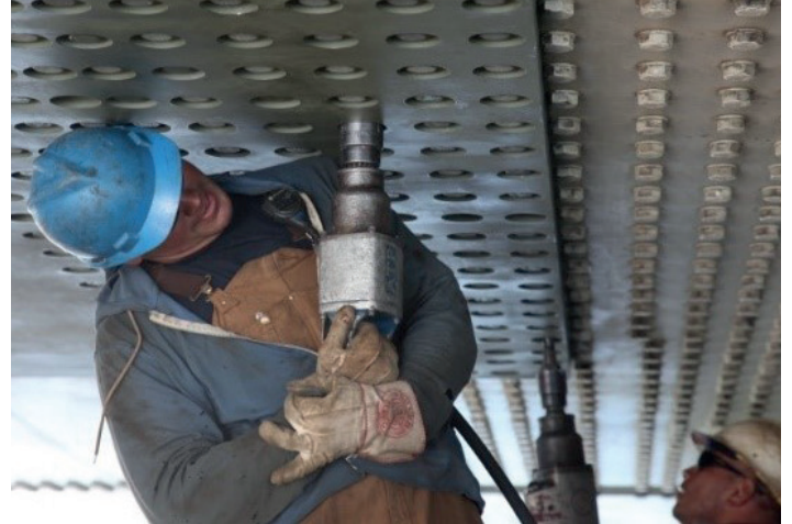
Traditionally bolts on bridges are fastened with noisy impact wrenches and slow hydraulic torque wrenches.
