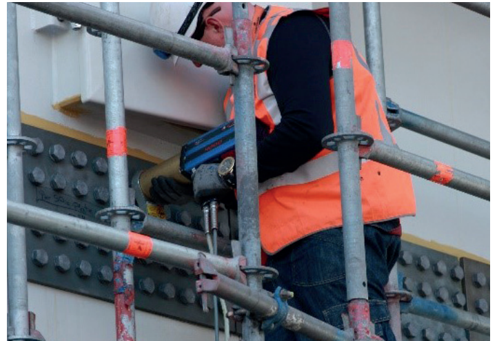
E-RAD 3400: on this particular bridge more than 4.000 bolts had to be fastened at 2.200 Nm.
