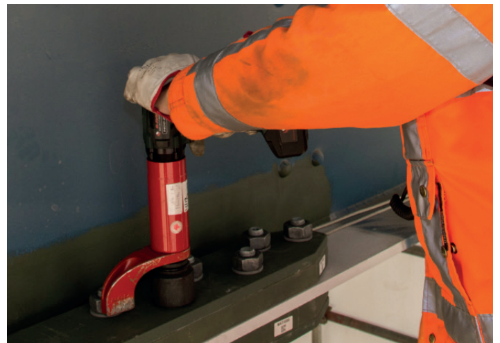
A B-RAD on one of the connecting plates. Thanks to the use of fast and accurate B-RAD tools the emergency repair was finished, and the bridge was reopened for heavy traffic, more than 2 weeks ahead of schedule. This drastically reduced the economic damage caused by the forced shutdown of the bridge.
