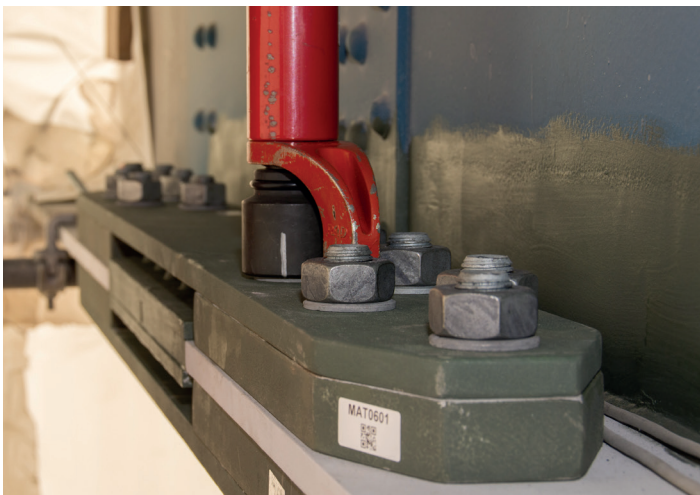
For an emergency repair on a bridge on one of the busiest highways in the Netherlands, thousands of bolts on specially made connecting plates were fastened with the torque and angle method. A large number of B-RAD tools were used for this job.
